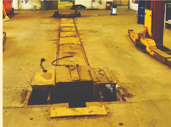
Replace two lifts, repair concrete floor, install epoxy floor.
