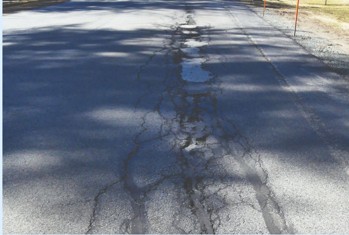
Reconstruct pavement at bus garage with heavy duty asphalt.
