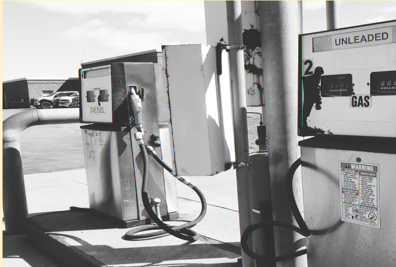
Replace fuel dispensing system at bus garage with modern, efficient system.
